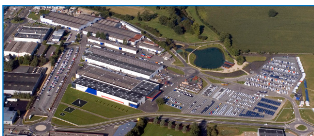
Gruau Group Headquarters Laval, France
